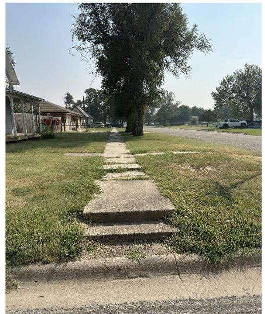
Poor sidewalk condition, non-accessible
